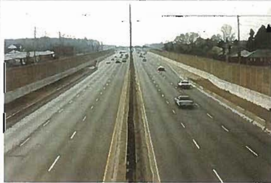
Figure 17. Reflective noise paths due to a single barrier
